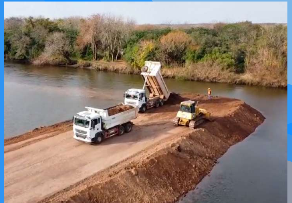
Santa Lucía's dam being built
